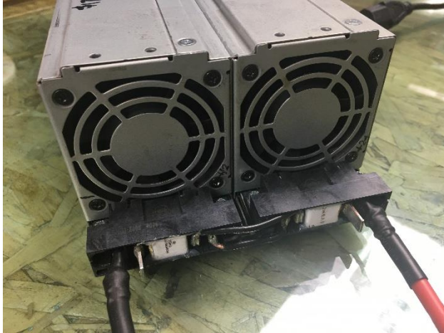
Figure 10 – Finished Connection at Power Supply
